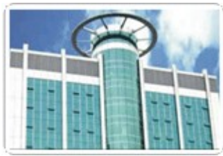
Guangdong Government Office Building
