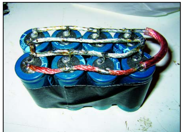
Like this. The loudspeaker cable has been stripped and well tinned at the places where the capacitors are soldered to it.
