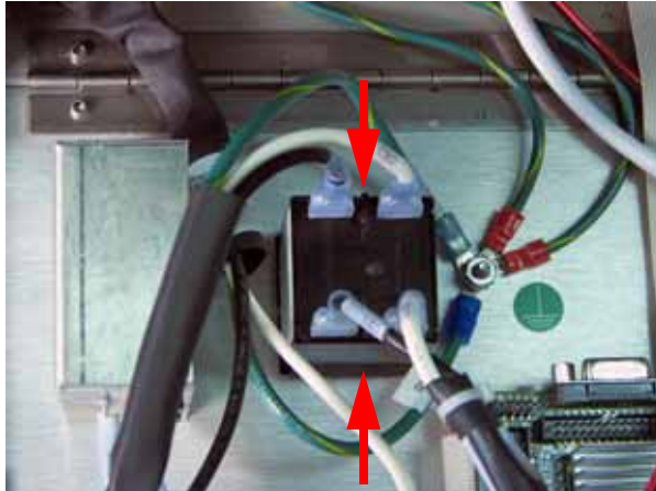
Figure 4-72: Removing the circuit breaker
