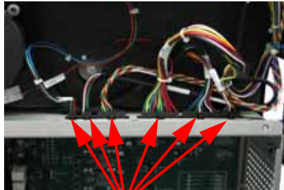
I/O Card cable locations
