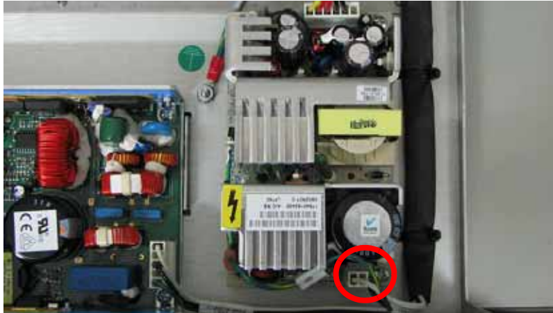
Figure 4-87: Power input cable location
