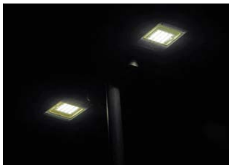
Figure 6. Night view of newly installed LED street lamps in the author's home town.
