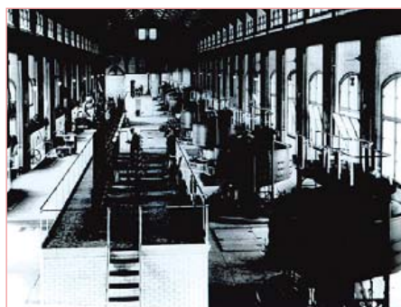
Figure 2. The hydro-electric power plant in Niagara Falls (1985).
