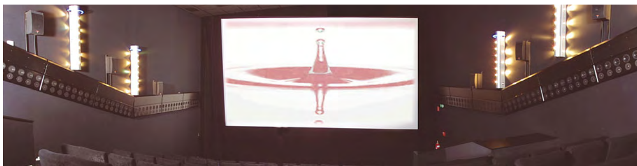
Figure 12. A wave field synthesis system in the 'Linden Lichtspiele' cinema in Ilmenau. The system has over 192 separate channels. (Photograph courtesy Fraunhofer IDMT/Ingo Herzog).
