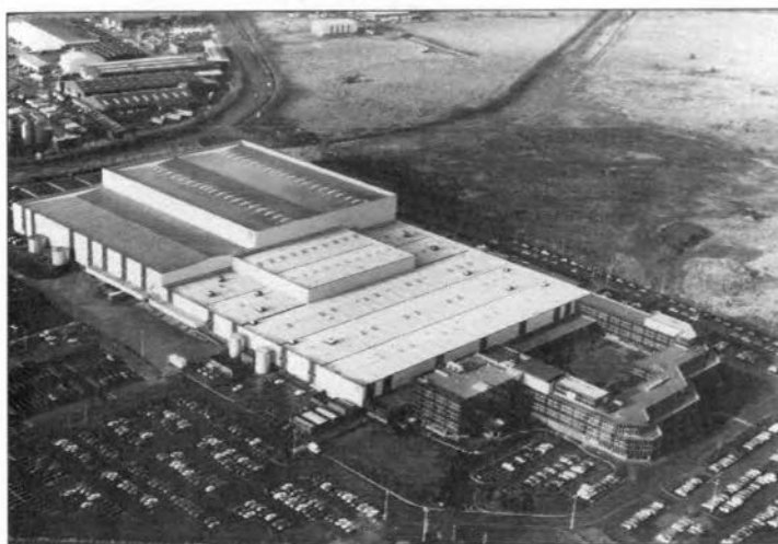
The RS Components headquarters are housed in a 75,000 m 2 (equivalent in size to ten football pitches) warehouse and office complex in Corby, Northants, England. Over 10,000 orders are processed at terrific speed every day at this location, including orders for the 'retail' branch of RS Components, Electromail.
