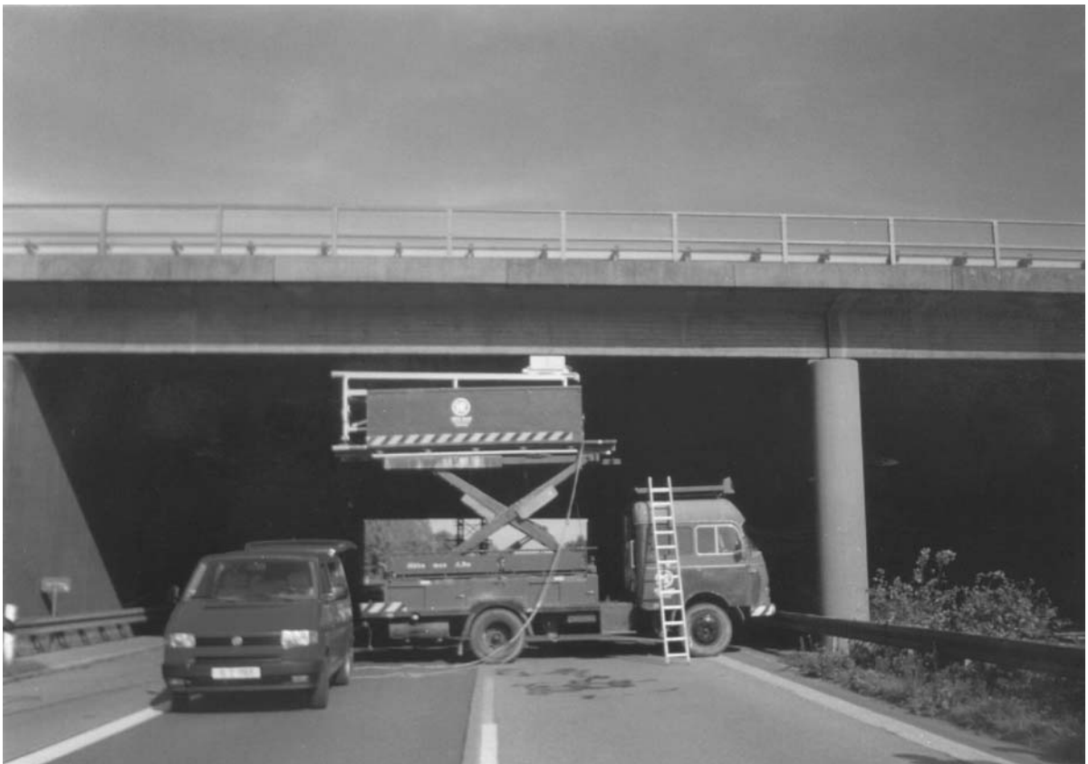
Figure 3 Inspection of a German highway bridge using a SQUID system.
