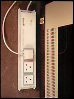
...the mains power supply to a PBX telephone exchange
